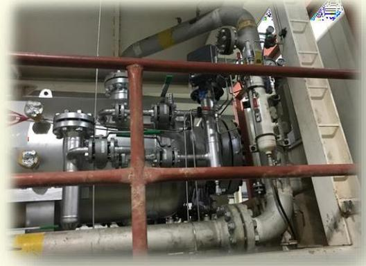
**Project: 1440PSI well test Separator Package Trailer mounted**
